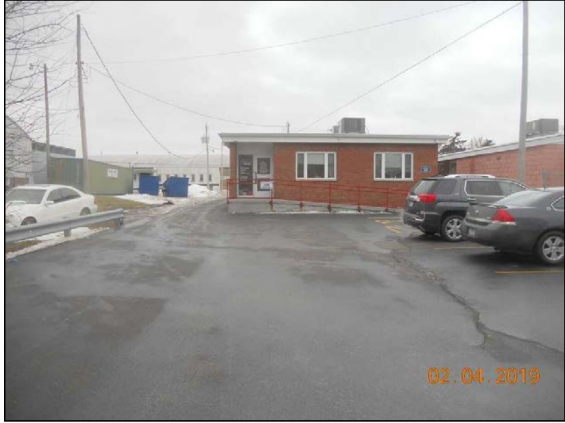
Rear of Subject
